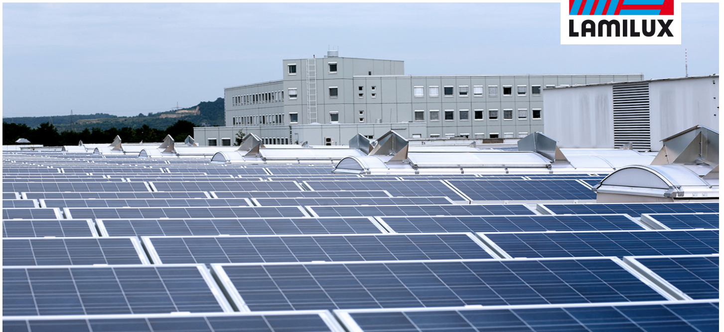
Schneider Electric, Regensburg, Germany
